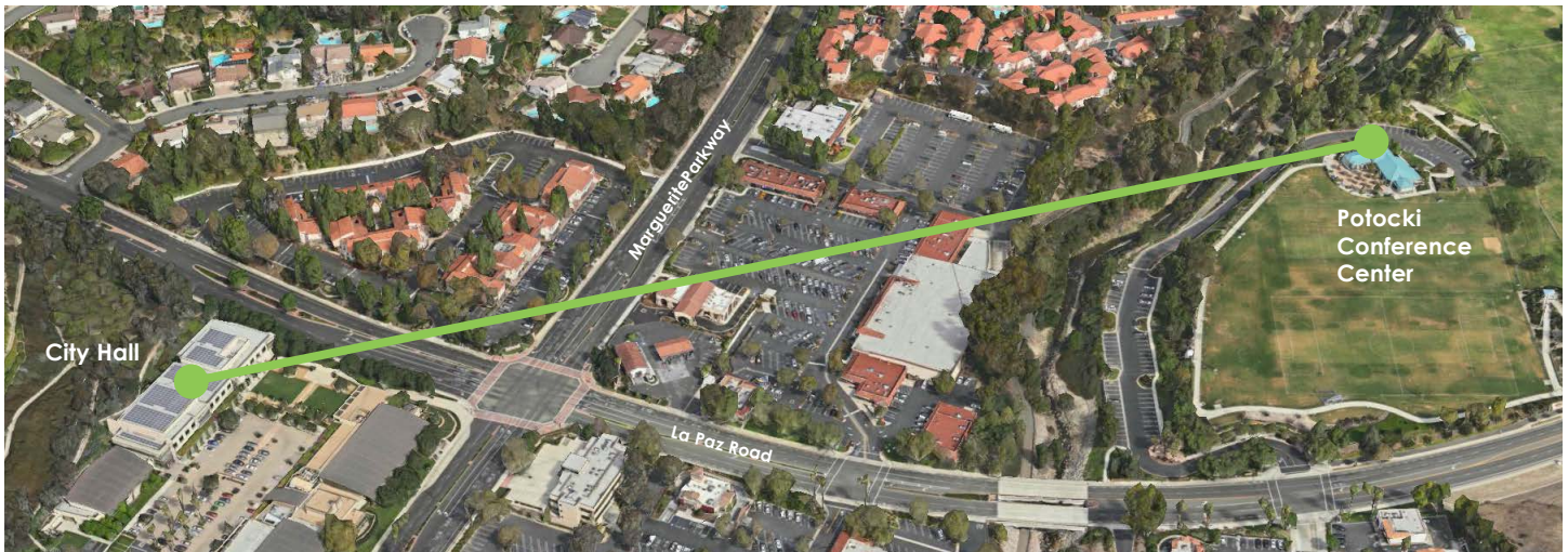
Mission Viejo's HaulPass V60s wireless broadband 600-meter connection from the City Hall data center to the Potocki Conference Center.
